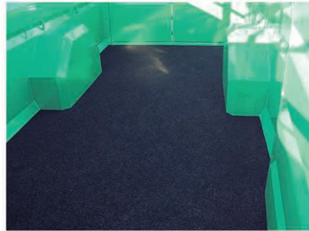
PISO CUBIERTO DE RESINA / FLOOR COVERED IN RESIN
